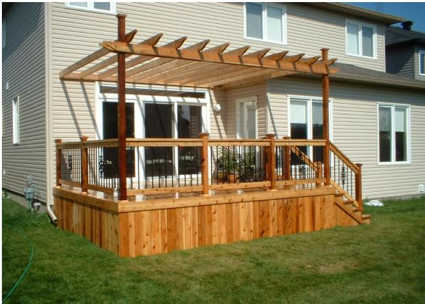
**Permit:** A permit is required for decks adjacent to or attached to the house and with a walking surface more than 600 mm (24 in.) above the adjacent grade, and If the deck is elevated and provides a principal access to a building.
